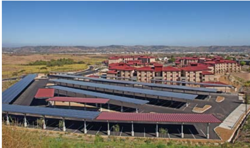
Atop a parking garage near one of the living quarters is one of the many photovoltaic arrays at MCB Camp Pendleton.
